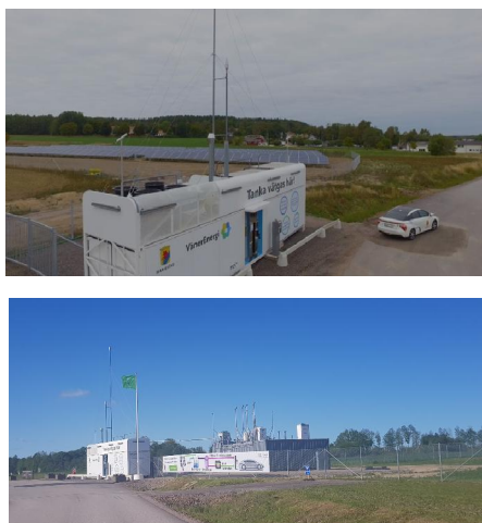
Figure 1 The off-grid solar hydrogen refueling station in Mariestad, Sweden. The PV park (top) supplies all the electricity needed to produce hydrogen. [Photo courtesy of Nilsson Energy].
