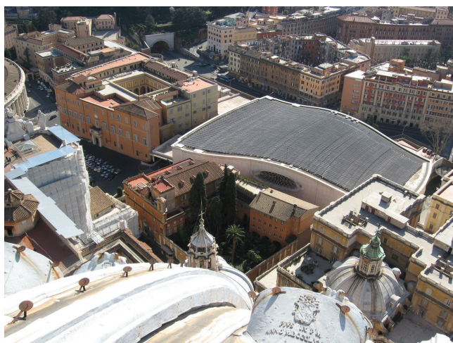
Figure 1. The photovoltaic array on the rooftop of “Paul VI” Audience Hall in the Vatican City. Image reproduced under the terms of the Creative Commons Attribution 3.0 Unported license. [17] Copyright 2008, Carsten Möller.
