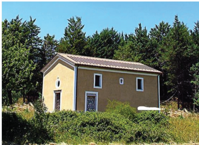
Figure 5. A 3.024 kWp solar array in PV tiles comprising the rooftop of Cappella dell'Incoronata, Cassano Irpino, Italy (Photo reproduced with permission, courtesy of FotoSun).
