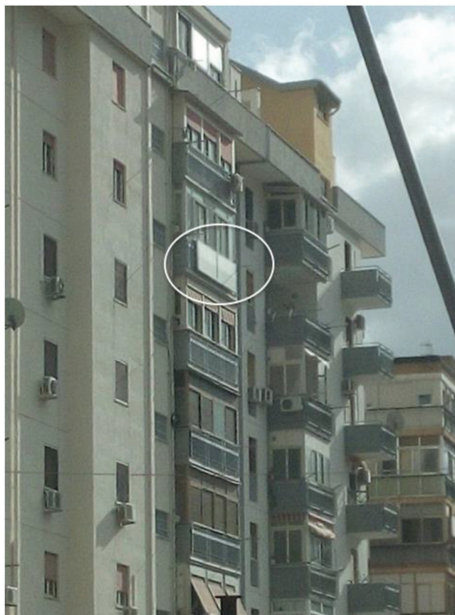
Figure 8. Custom-size solar air thermal collector integrated in the balcony of a residential building in Palermo, Sicily.
