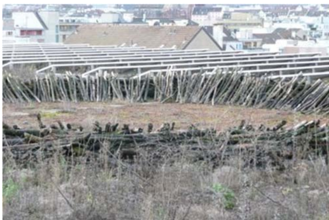
Figure 3. The solar green roof completed in 1999 on the Hall 1 of Messehalle Basel (after addition of organic matter and woody debris in 2008). (Photograph of Jim Labbe, reproduced with permission. [17] )
