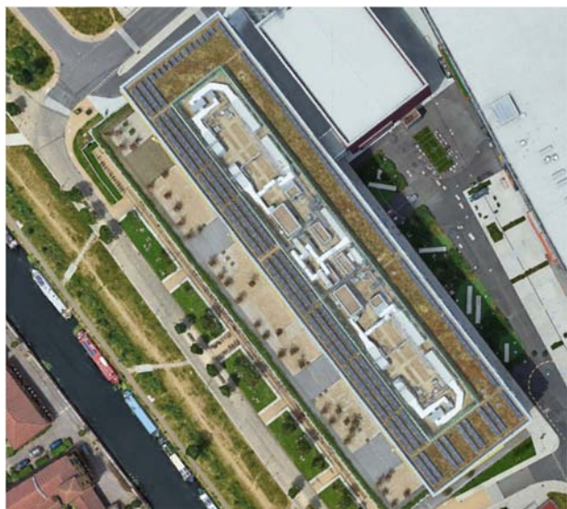
Figure 8. The four-storey London Olympics International Broadcast Centre hosts a 2500 m 2 green solar roof whose habitat attempts to mimic the open habitat of the Thames river corridor (photographs from Google Earth).
