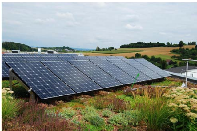
Figure 1. The green roof provides a superimposed load. There is no roof penetration, thanks to the superimposed load principle (photograph courtesy of ZinCo GmbH).
